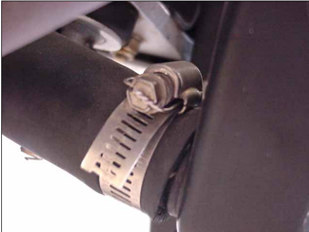
Safety tie the hose clamps
