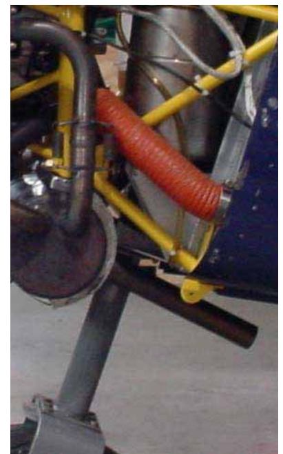
Tail pipe on left side of nose gear.
