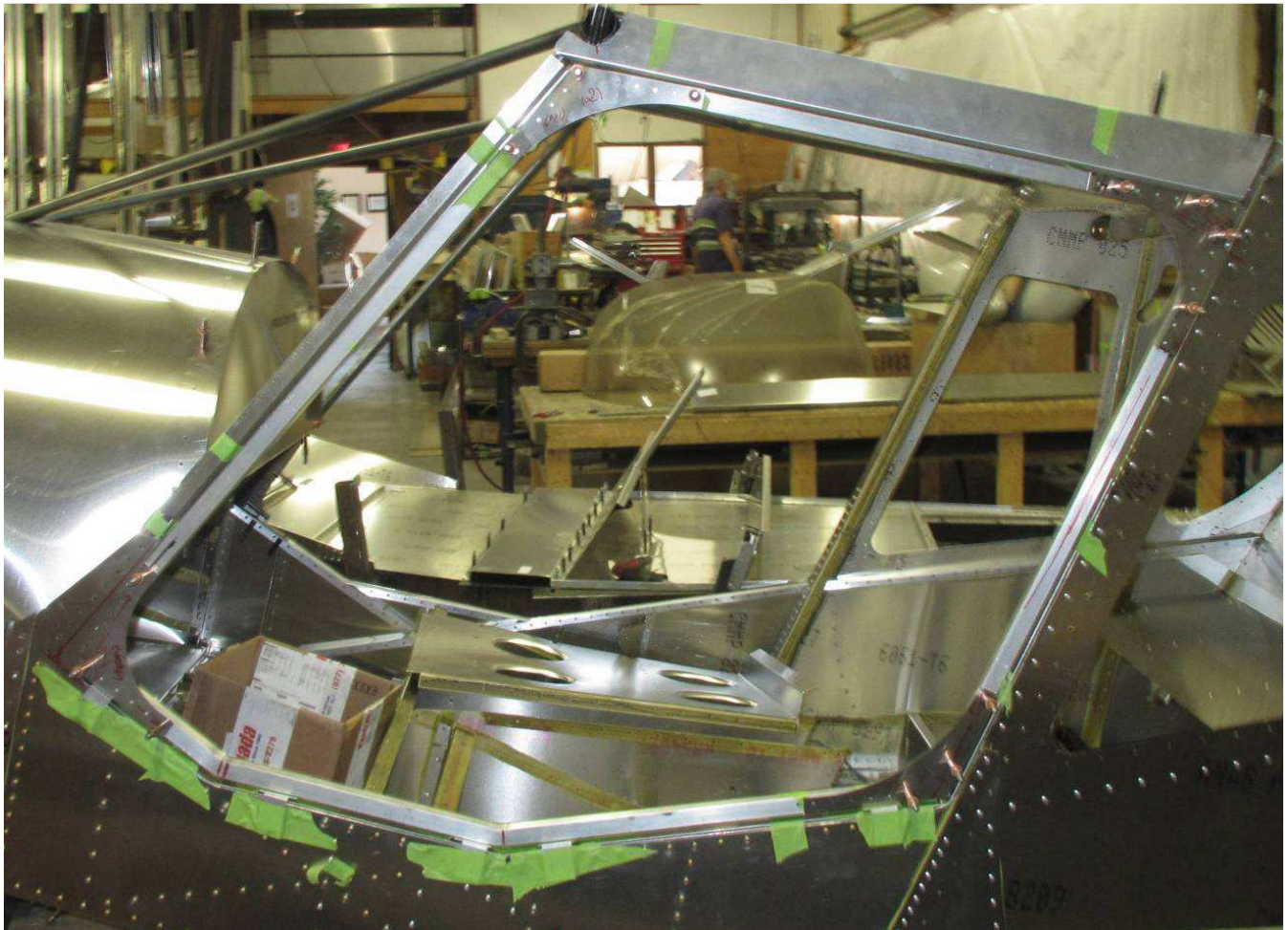
The 4 O/B gussets are now clecoed to the frame
