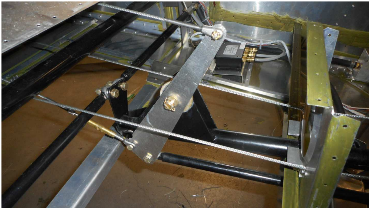
The rudder cables run in the space between the control mixer 75C1-6 and the horizontal flaperon control rods 75C2-1
