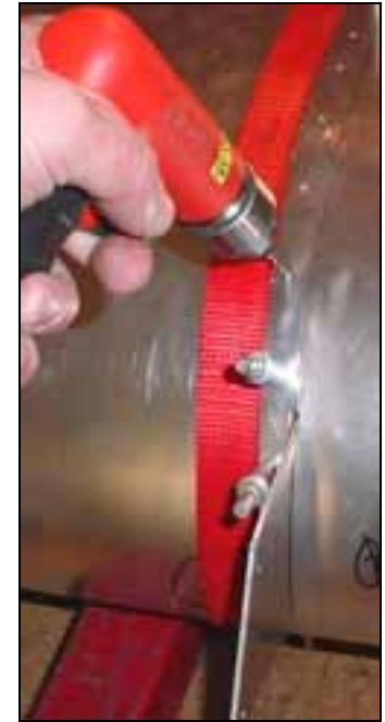
Start drilling at the front and work your way back.
