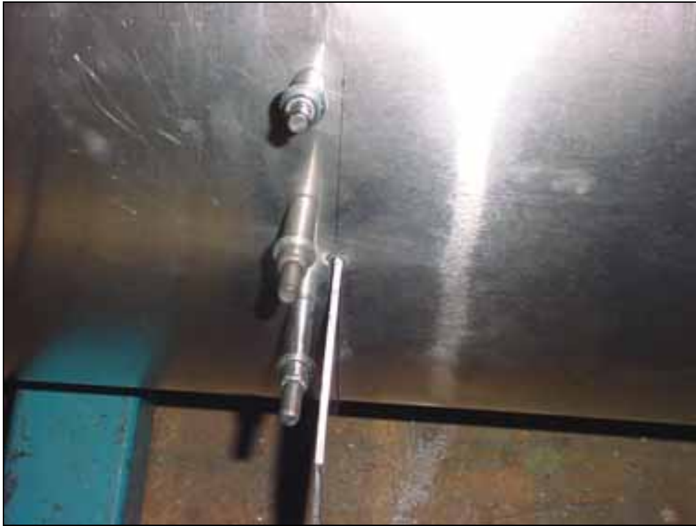
Layout the rivet line for the rivet line through the bent L angle on the I/B side of the slat supports 7V4-5
