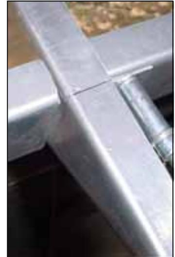
The inboard channel is in line with the channel on the outboard side of the rib.
