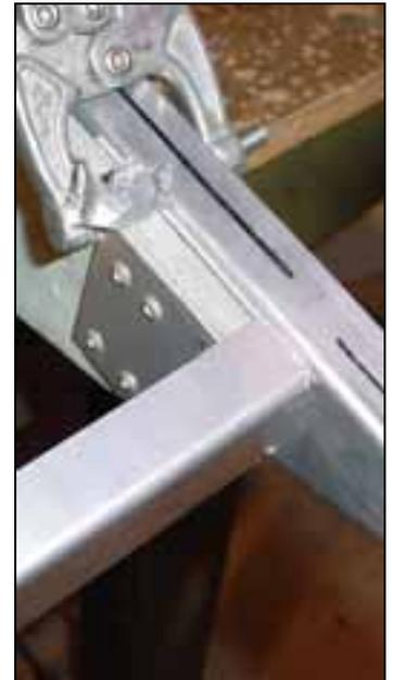
Slide the bend end of the rear channel over the end of the template. Bend flange fits between the side of the rib and the template.
