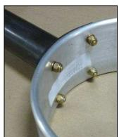
The holes can be opened up to the correct size and bolted together.
