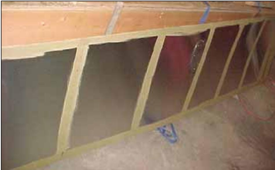
Primer applied over the rivet line (inside surface only).
