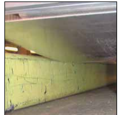
At rear rib #1 the 2" steel beam does not fit between the workbench and the skin.
