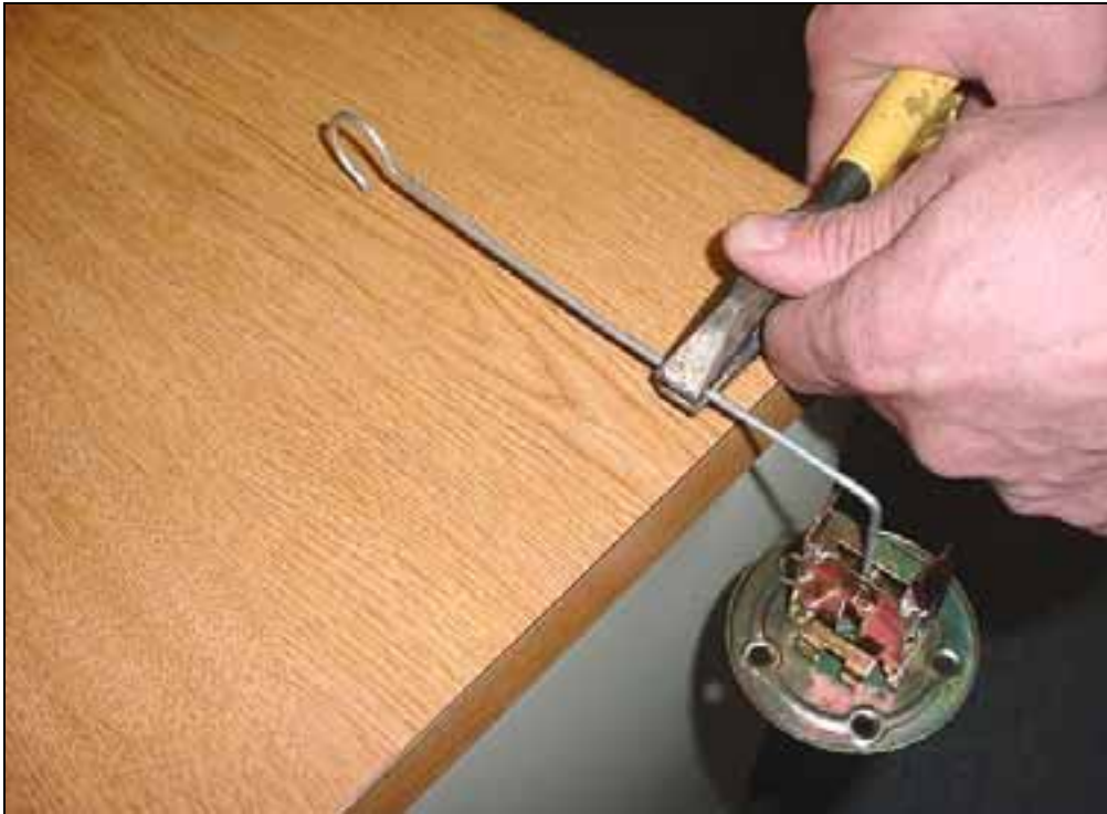
Position the pliers on the sender side of the 65mm mark.
