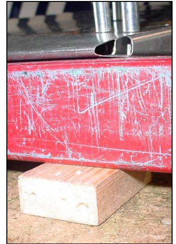
Spacer under aft bottom corner.
