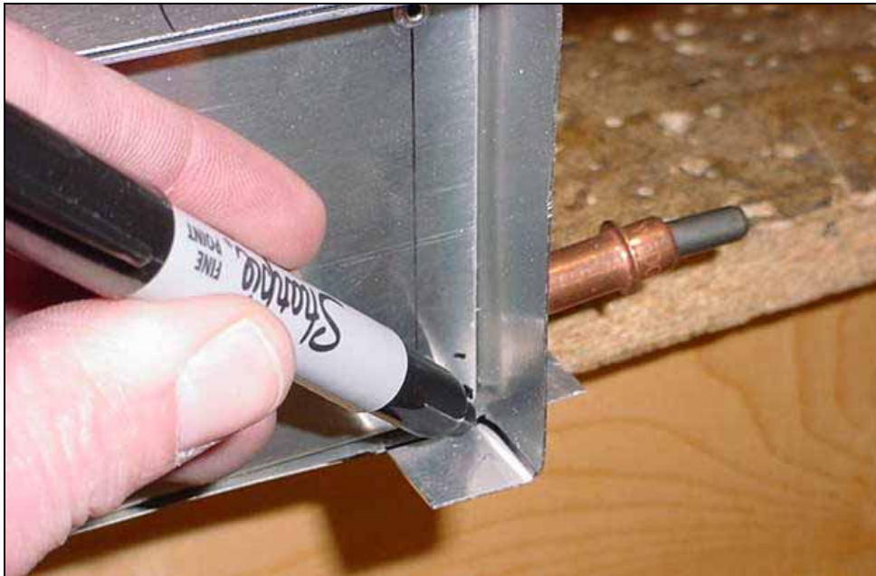
Trace the spar on the flange.
