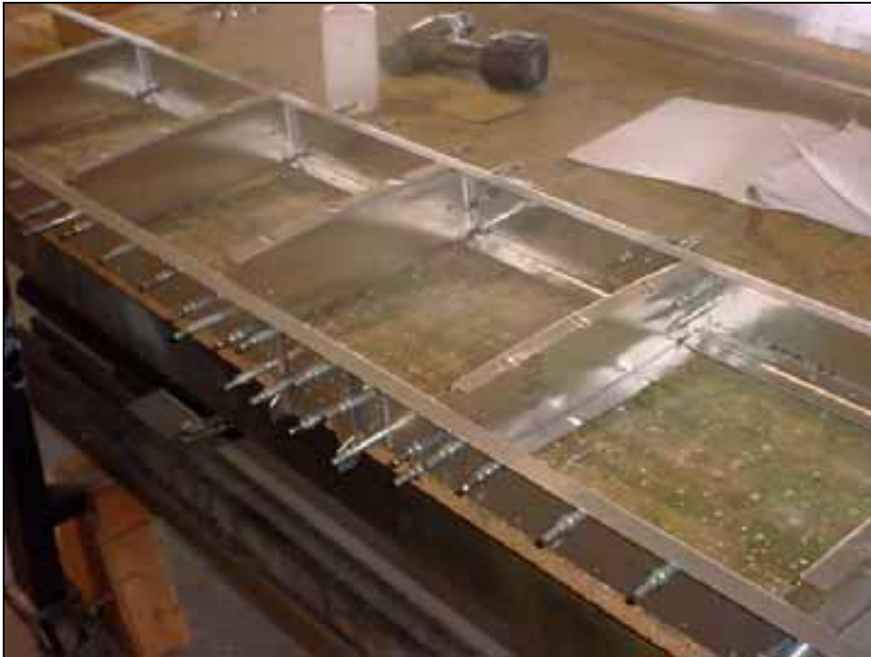
Drill & Cleco ribs to spar.
