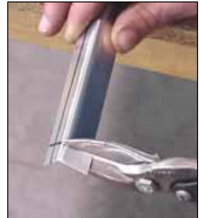
Final cut: start on one flange and keep snipping around radius across to the second flange.
