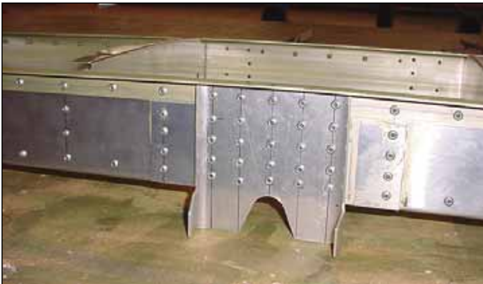
Ref holes in top and bottom doublers: wait to open up the holes to #20 until after the center ribs are installed.
