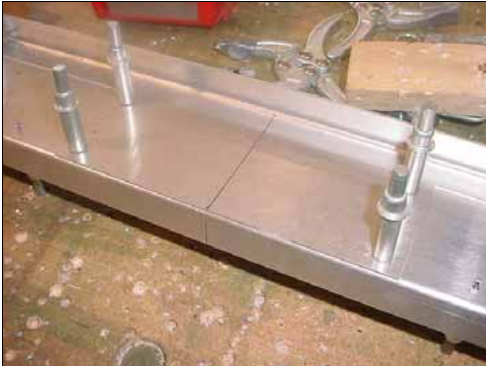
Layout the center line on the rear spar attachment 6T2-3.
