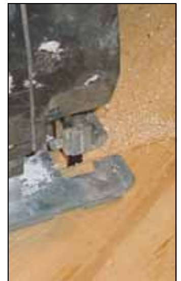
Try to have a smooth cut with minimum cuts on the outside of the line.
