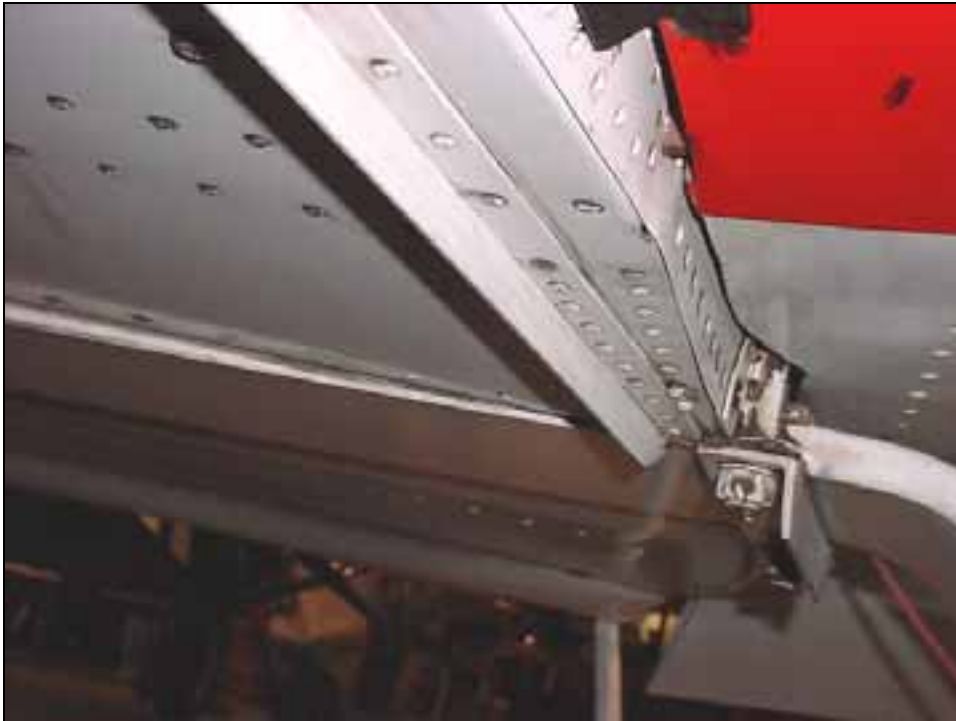
Bottom view of the rivets in the Gusset 6B10-4, transition to the bend in the cabin floor skin
