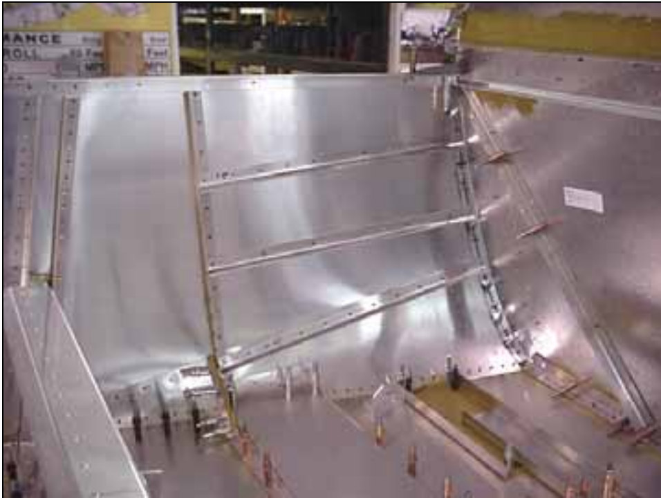
Inside view of left side.
