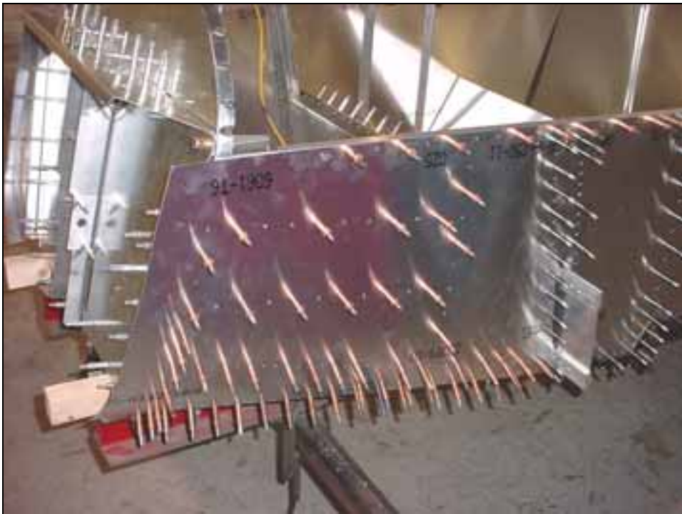
Finish drilling the top edge of the side skin to the Longeron 6B11-2, the first rivet is 140mm from the firewall rivet line (to allow for the overlap of the Forward Top Skin 6C1-4)
