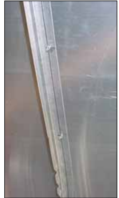
First layout out the location of the horizontal L angles down the vertical L angle, Pre-drill the intersection holes with pilot holes.
