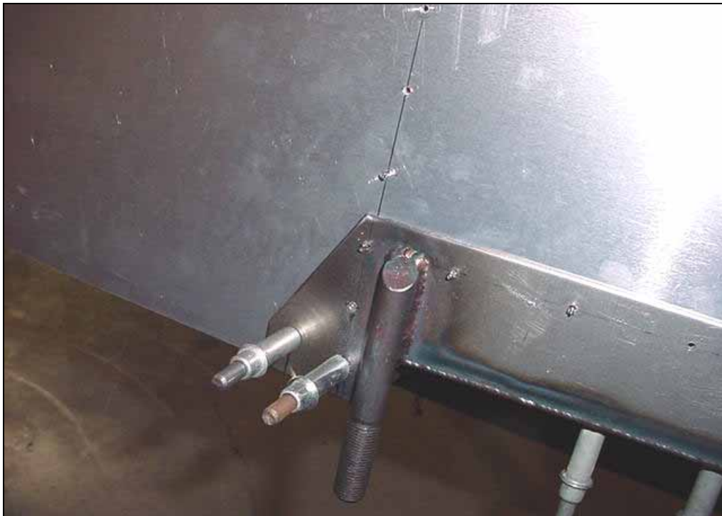
Drill the two aft bottom AN3 holes through the bottom longerons 6B2-3
