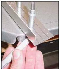
Trace the bottom of the firewall on the stiffeners and trim the stiffeners flush to the bottom edge of the firewall.
