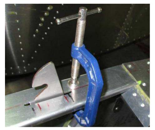
Check that the latch is pushed against the rivets in the side skin.
