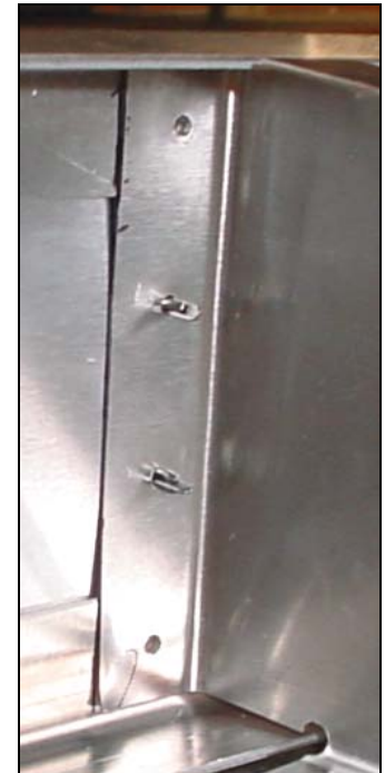
View of rib flange.
